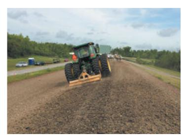
**Site Preparation:** Grade and compact the failed slope and remove objects that would prevent ARMORMAX from making direct contact with the soil. Excavate a trench at the crest and toe of the slope.
