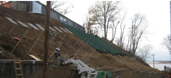
INSTALLATION ARMORMAX was installed, complementing the use of soil nails
