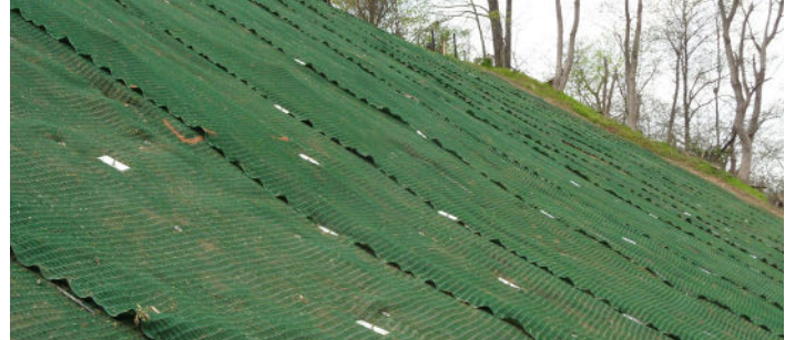
SOLUTION ARMORMAX and soil nails stabilize against surficial and global failure
