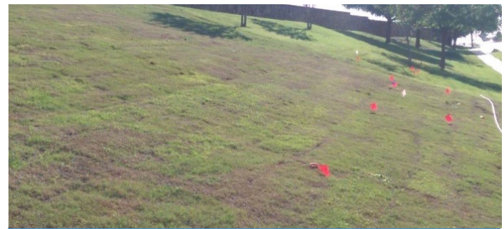
PERFORMANCE Vegetated engineered earth slope stabilization that is more aesthetically pleasing that also provides water quality improvements
