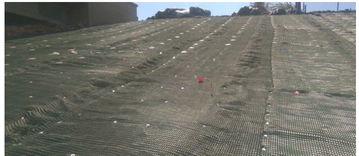
SOLUTION ARMORMAX® 75 Engineered Earth Armoring Solution for roadway and railroad bridge embankment stabilization
