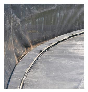
The floating cover is installed on top of the liner, after installation is finished, the manure/effluent is pumped between the liner and the floating cover. Floats with outlets under the cover keep the membrane floating, even after heavy rain fall. As a cover, high UV resistance of the TenCate Nicolon<sup>®</sup> C119/800 membrane is one of the most important properties.
