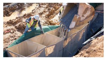
**SOLUTION** SCOURLOK units were filled with in-situ soils, eliminating the cost of importing fill material to the jobsite
