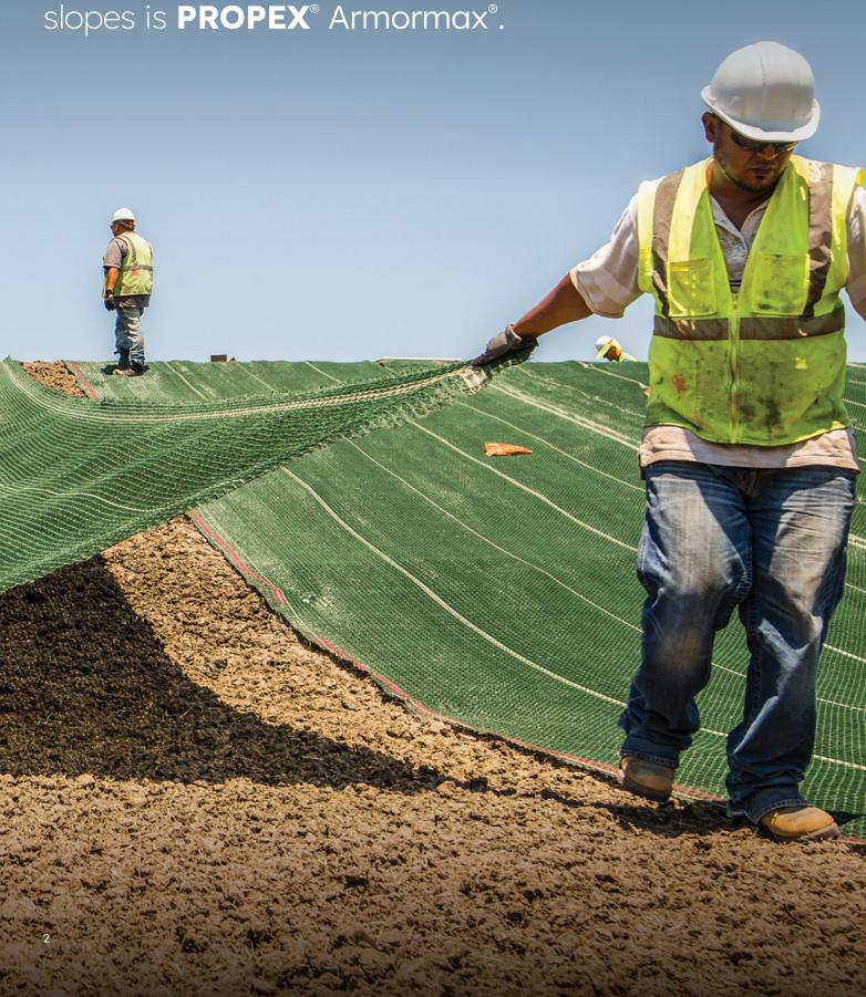
PROPEX Armormax is composed of High Performance Turf Reinforcement Mat (HPTRM) and Engineered Earth Anchors that work together to lock soil in place and protect against hydraulic stresses.
